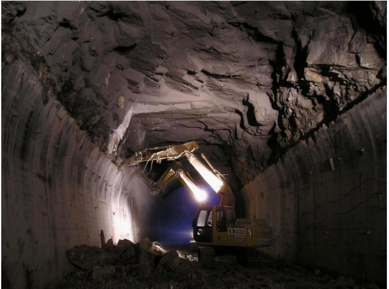
Construction work to raise tunnel clearances for the Heartland Corridor Project
