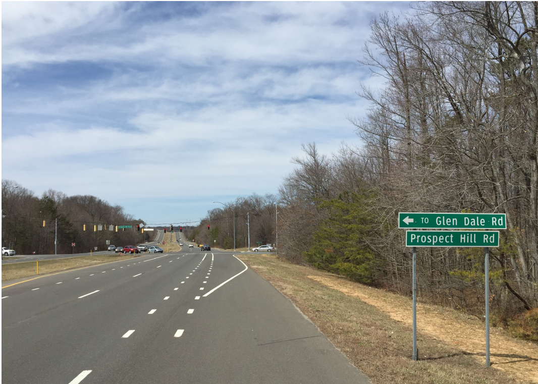
Figure 12-5: Shoulder Transition to Bike Lane at a Right-Turn Lane on a Rural Arterial
