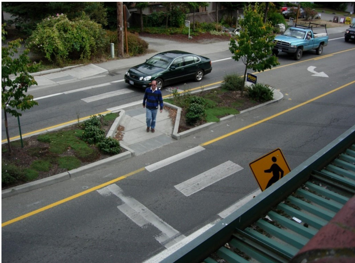
Figure 3-35. Angled Crossing Through a Median Island to Encourage Pedestrian Awareness of Traffic on the Roadway about to be Crossed
