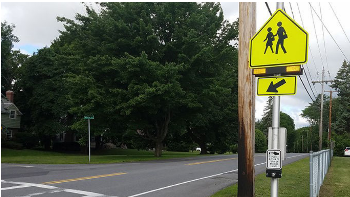
Figure 3-37. Rectangular Rapid Flashing Beacon Installation
